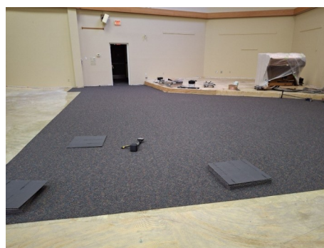
The new carpet tile being installed
