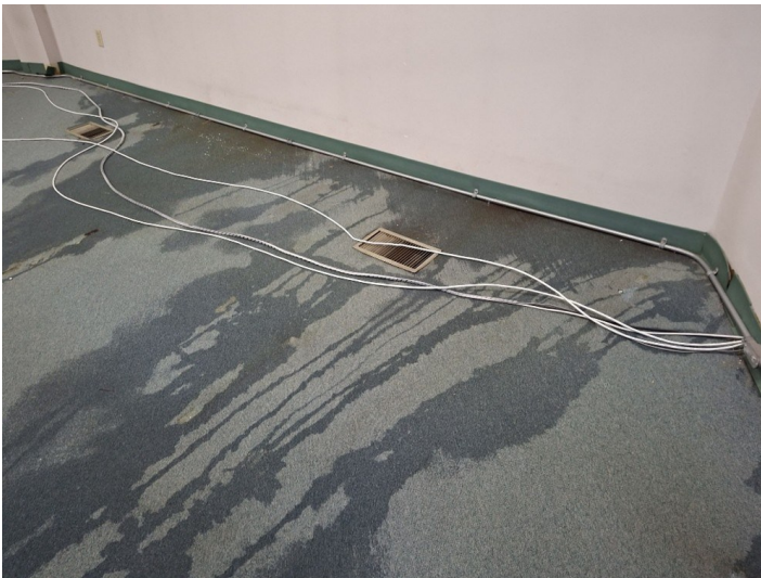
Leak at the back of the sanctuary after the hail storm
