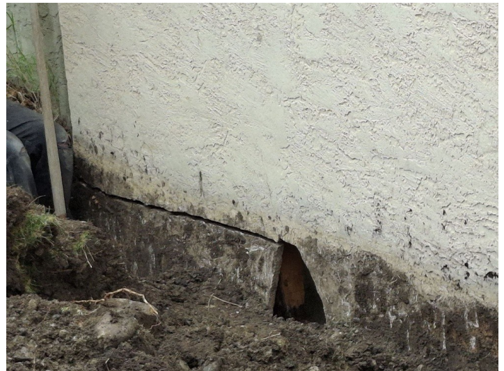
The source of the leak is uncovered
