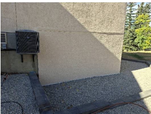
Repaired wall restuccoed.
